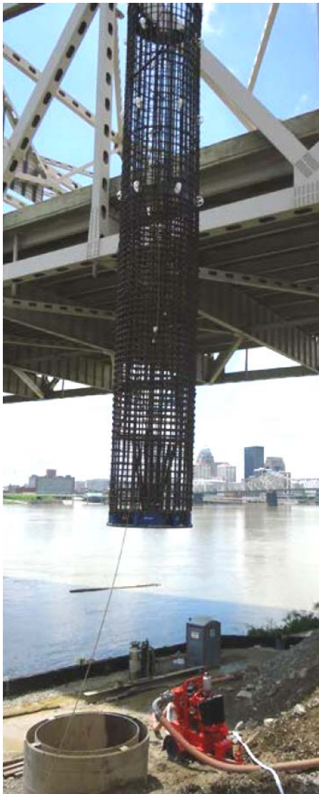
Reinforcement cage installation with O-cells
