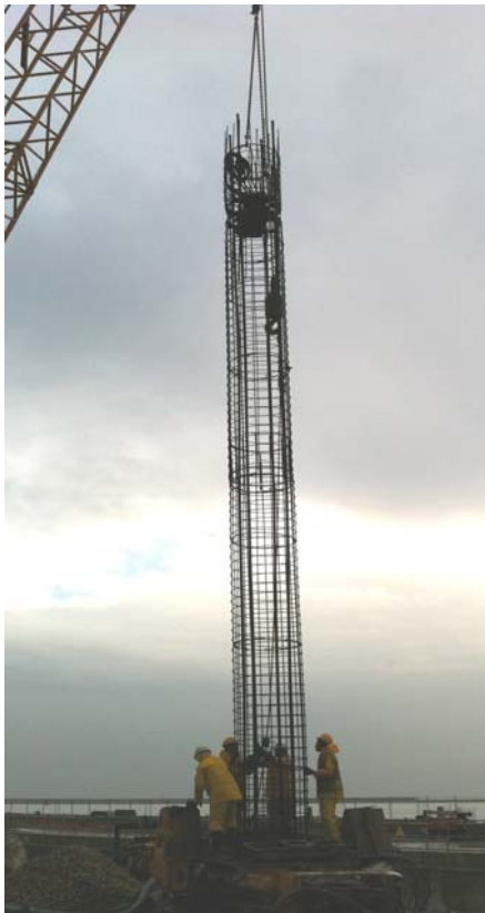
Installation of the O-cell cage
